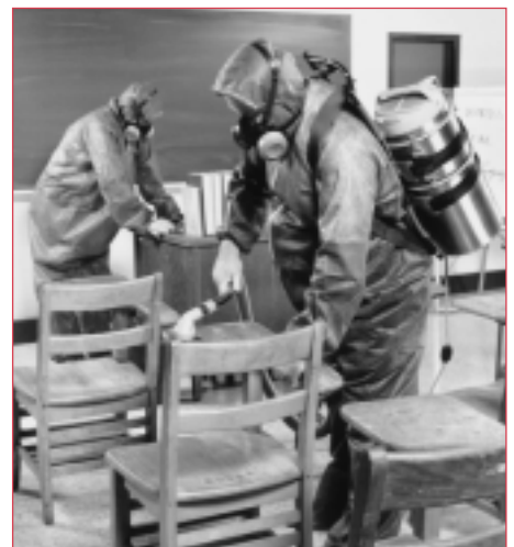
The Compact Vac being used by an AHERA team to clean a contaminated classroom.
